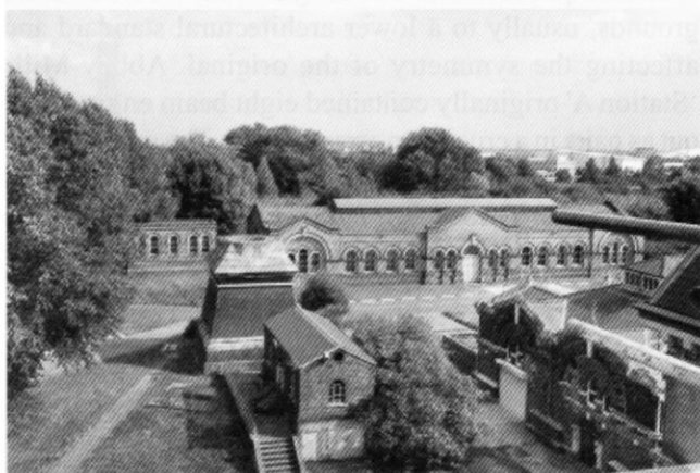
The base of one of the two chimneys demolished during WWII. Photo Nick Catford
